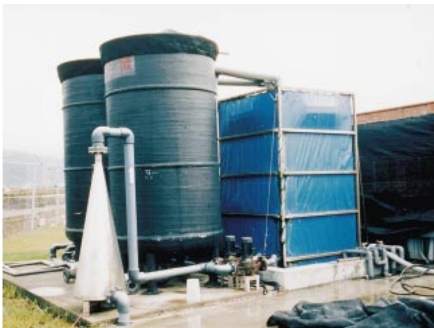
Fig. 1 Water treatment facilities for an super-intensive aquaculture system that boasts stable water quality and low water consumption.
